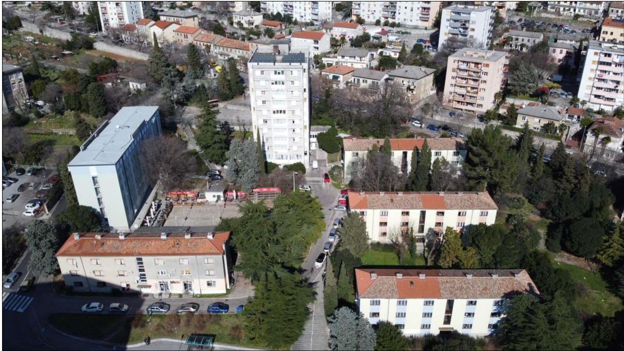
Picture 4. Student dormitory Ivan Goran Kovačić: pavilions 1, 2, 3, 4 and 5
