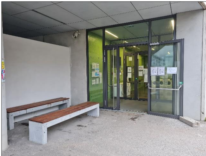
Pictures 19. Laundry room
